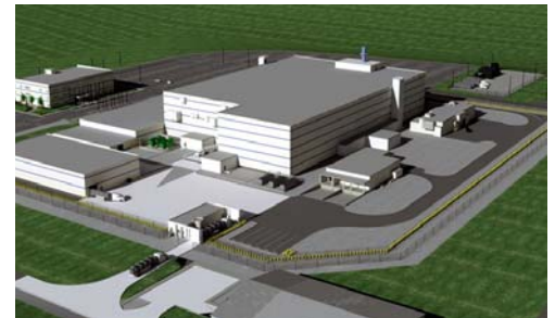
The National Nuclear Security Administration (NNSA)'s Mixed Oxide (MOX) Fuel Fabrication Facility.
