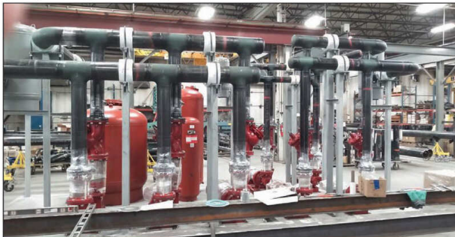
Harris' work on the 668,000-square-foot Heywood Bus Garage project included prefabricating a massive pump skid. The 21-foot by 10-foot skid weighing roughly 15,000 pounds houses the base-mounted pumps, expansion tanks, air separators and pot feeders for the chilled water, ground source water and heating water systems running the building. Photo: Harris.
